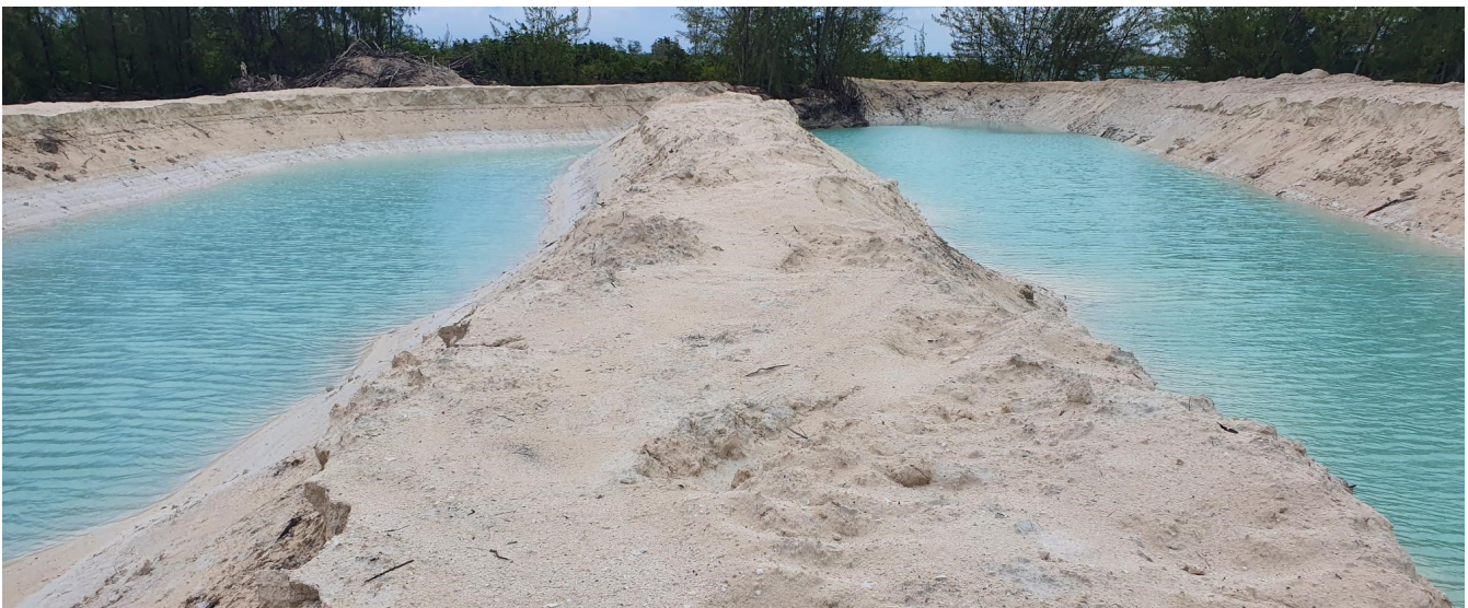
Project dewatering area
