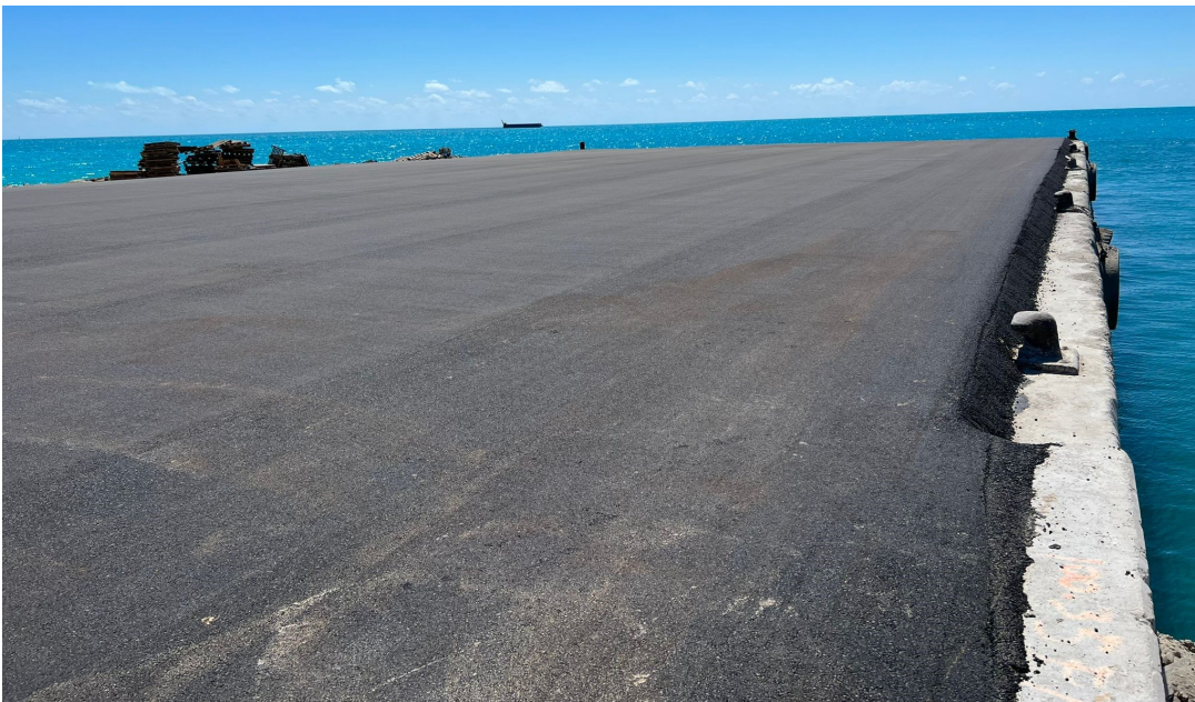
Newly pave bulkhead
