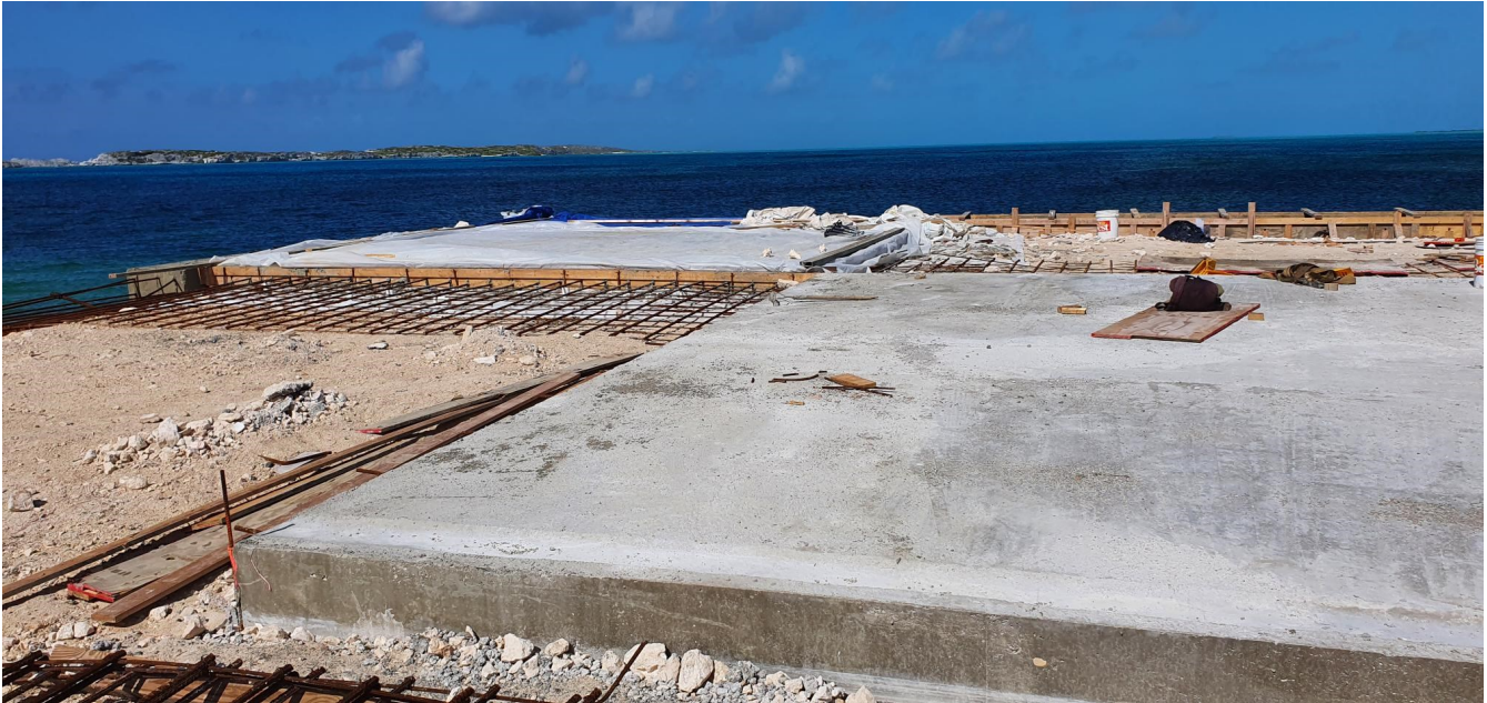
Bulkhead during construction
