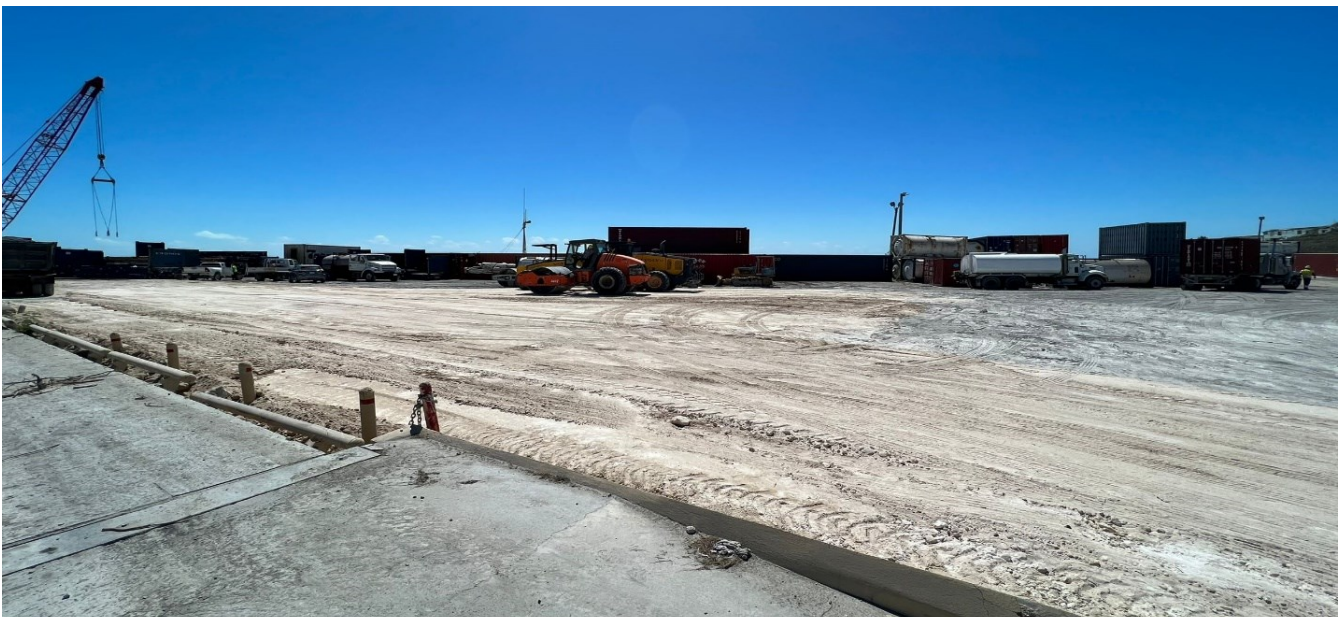
Earthworks in the main container yard
