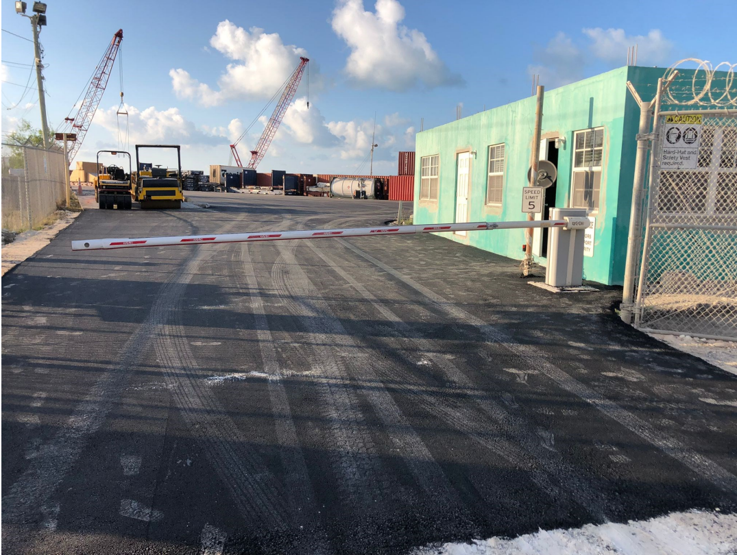
Newly paved port main gate
