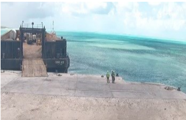
Vessel offloading at the new bulkhead, South Caicos
