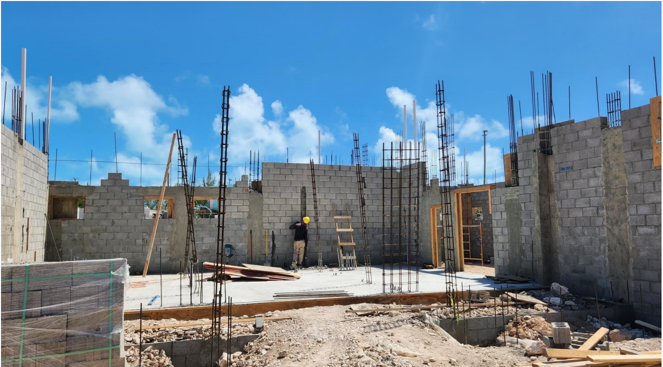
Construction of the first floor of the new office building
