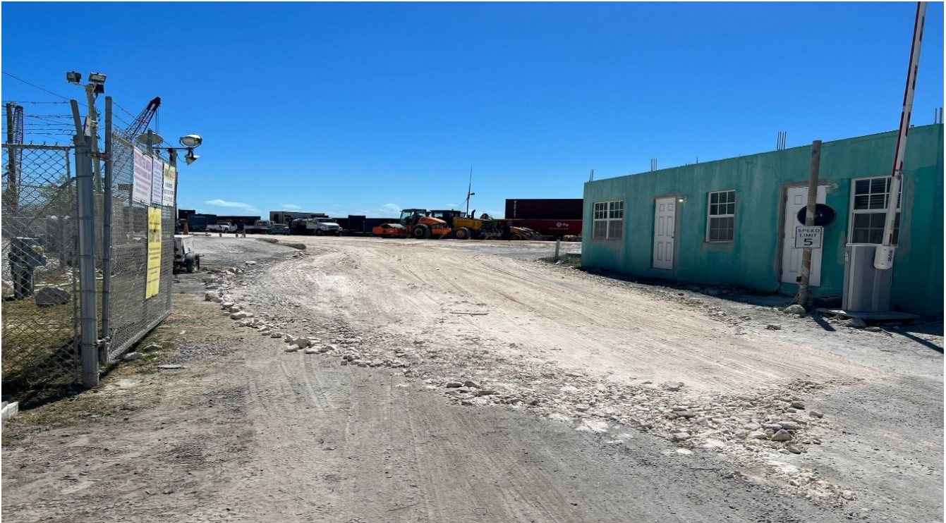
Earthworks at the main gate
