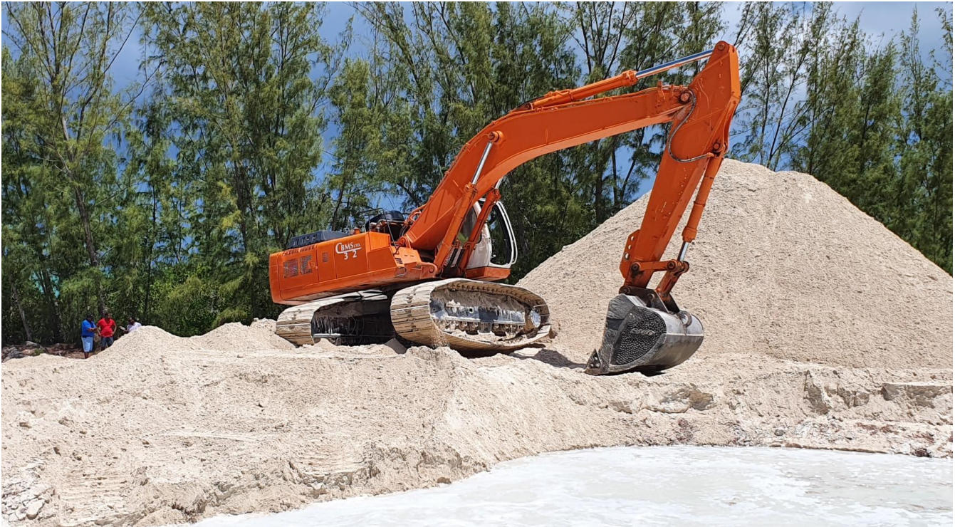
Stockpiled sand from dredging operations
