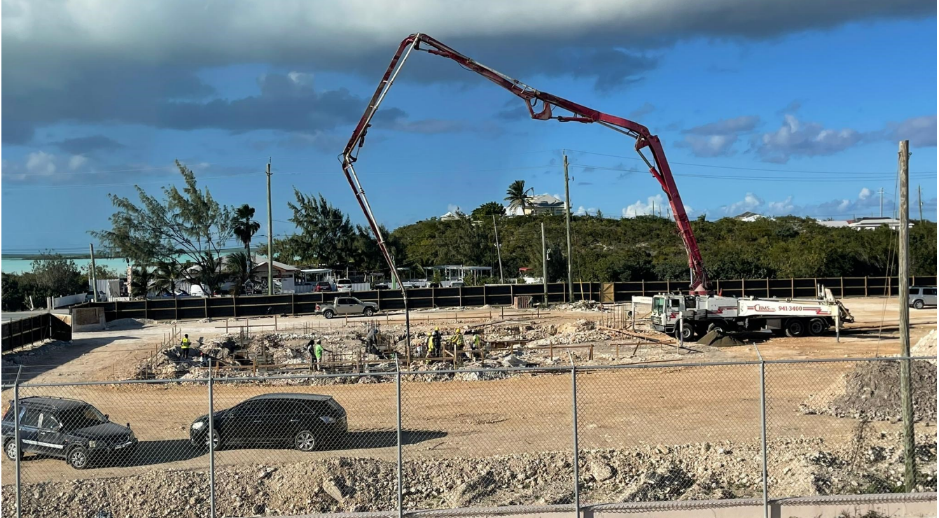
Pouring the foundation of the new office block
