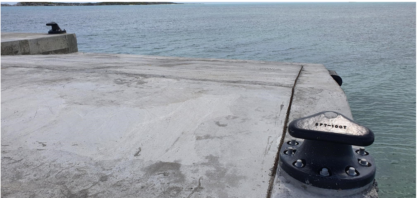
New 'Ro-Ro' Ramp included in completed bulkhead
