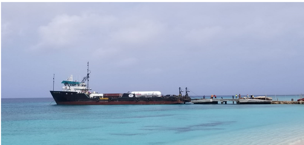
Offloading ISO tanks at recently constructed 'ro-ro' ramp South Dock, Grand Turk
