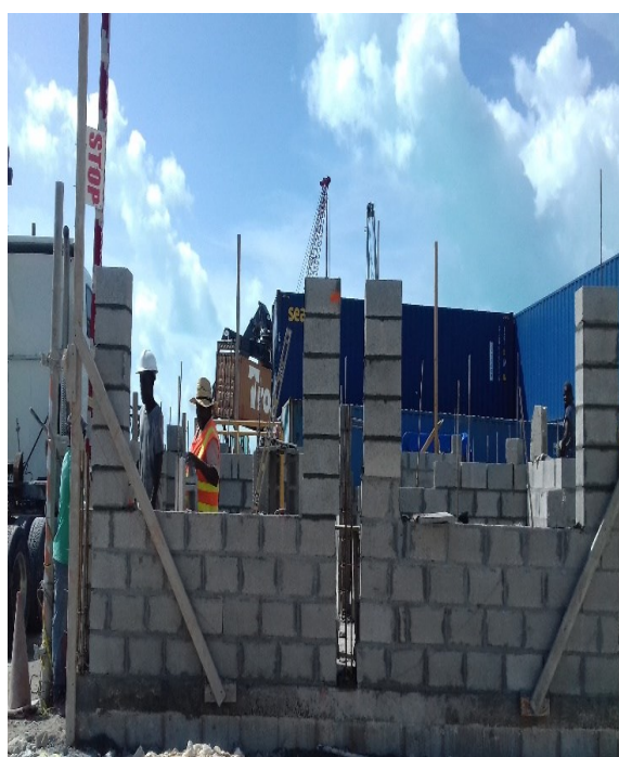
Construction of new Security Gatehouse, South Dock, Provo
