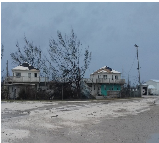
Hurricane damage at South Dock, Grand Turk
