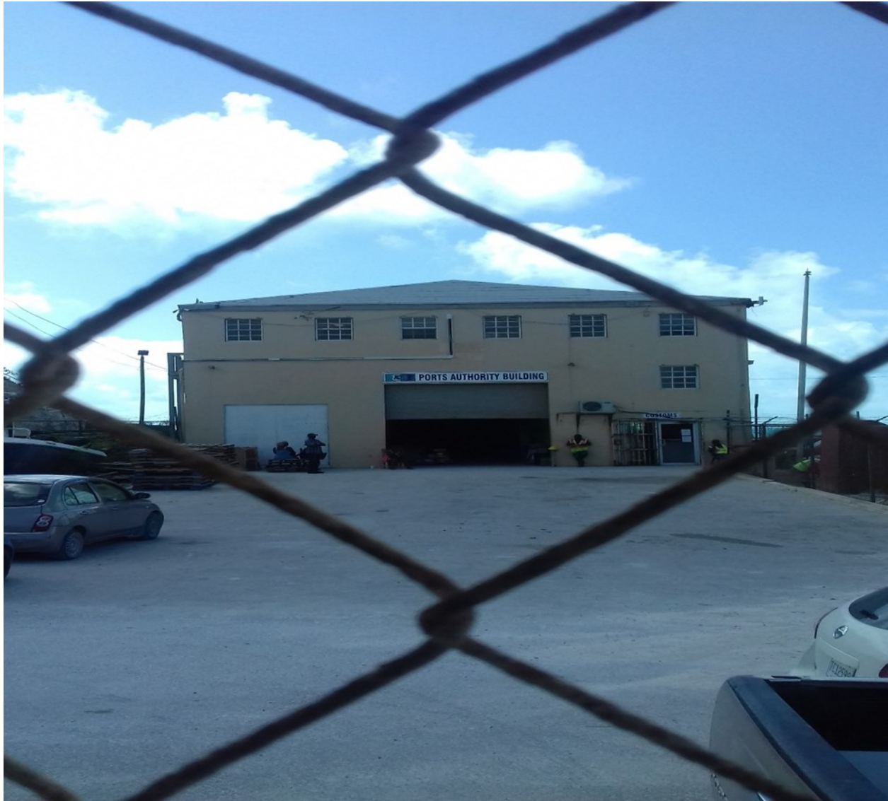
Ports Authority Office, South Dock, Providenciales
