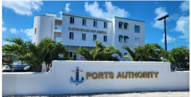
Completed Port Office Complex
