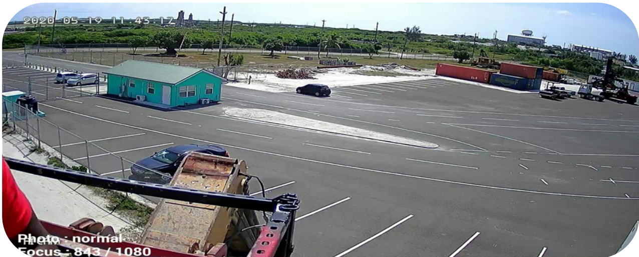
Completed, South Dock Pavement Project
