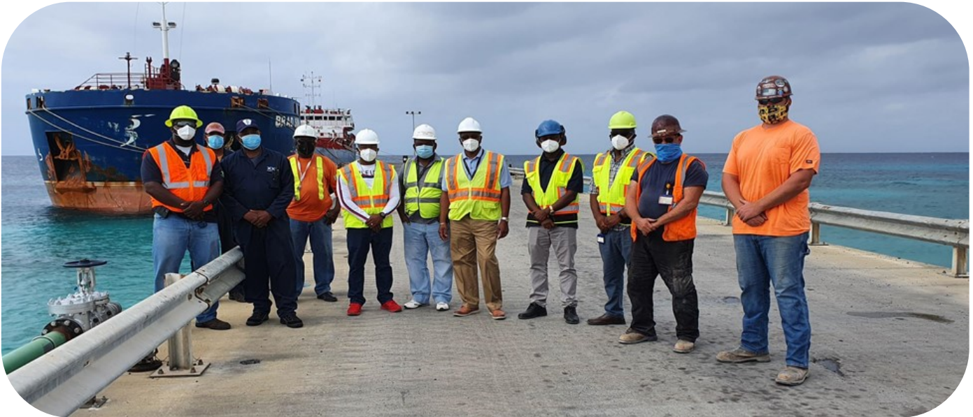
Commissioning of the new fuel pipeline
