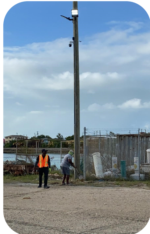
Installation of lights at South Caicos Port
